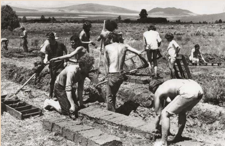
Making adobe bricks in 1968 for the Dome .
