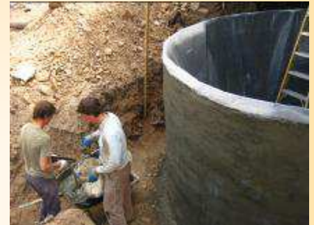
Working on the 5,500 gallon cistern
